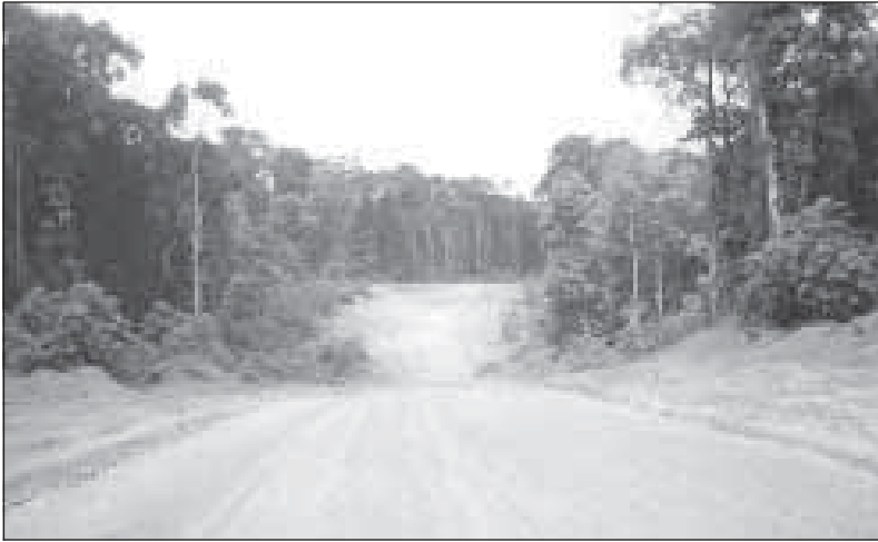
Timber road, south-east Liberia.
